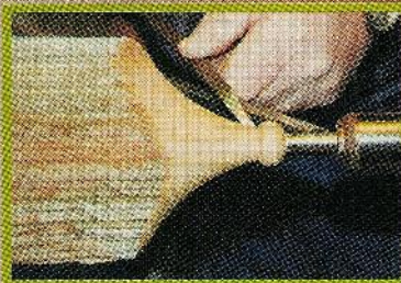
Fig. 8. After forming the bead detail, undercut the cove to bring it in line with the base of the bead.
