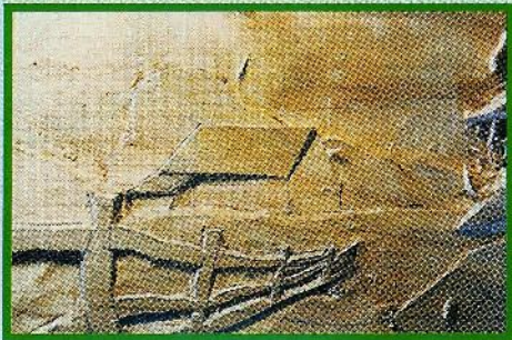
Fig. 7. Begin working on the barn roof and the lean-to.
