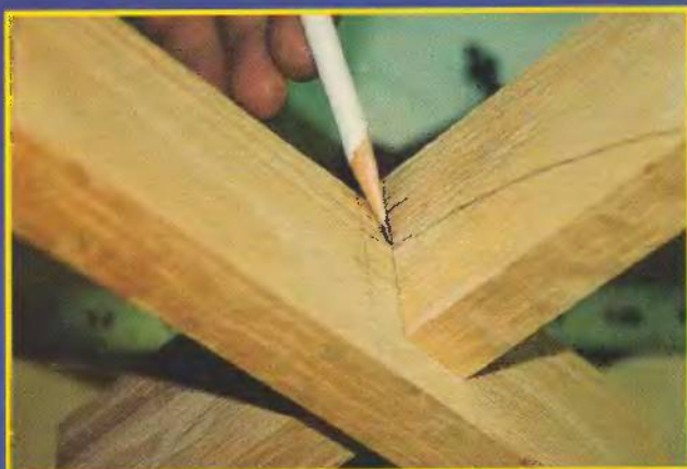
Fig. 4. Locating where the bottom of the mating half lap joint will be.
