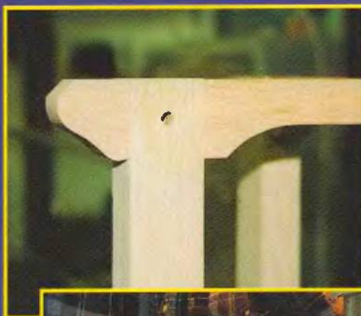
Fig. 7. The hole bored for the pin that reinforces the tenons (upper bridle joint shown). I located these holes by using a square to draw in the bottom of each tenon and then connected the corners of the square that was formed. The 1/4"-Dia. hole was bored in the center approximately 15/16"-deep.
