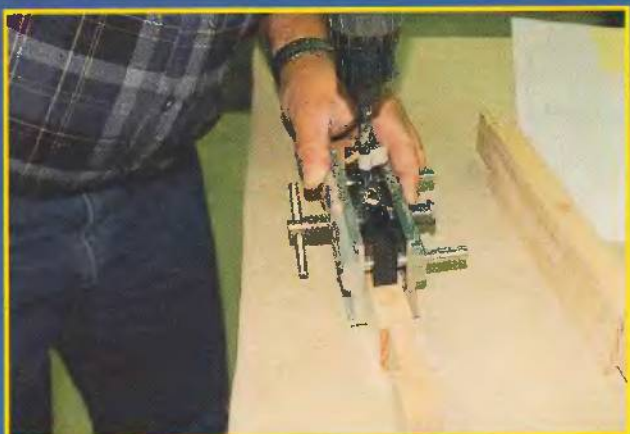
Fig. 5. Boring the locating pin hole in the top half of each set of rails. This hole will be deepened later on, after the stand is glued together.
