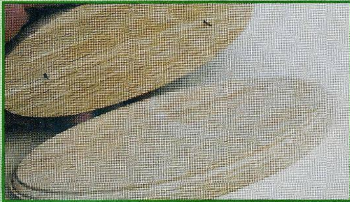
Fig. 1. Drill two small holes on either side of the bottom of the top base piece and put the finishing nails in the holes.
