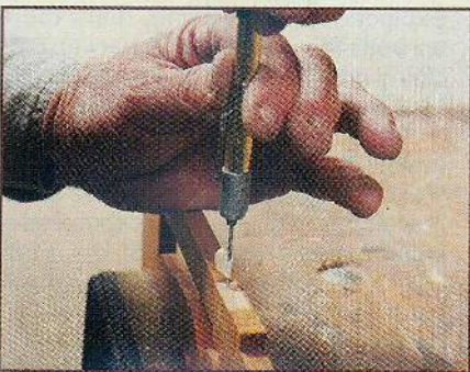
Fig. 5. Bore small diameter pilot holes for the hinge screws.
