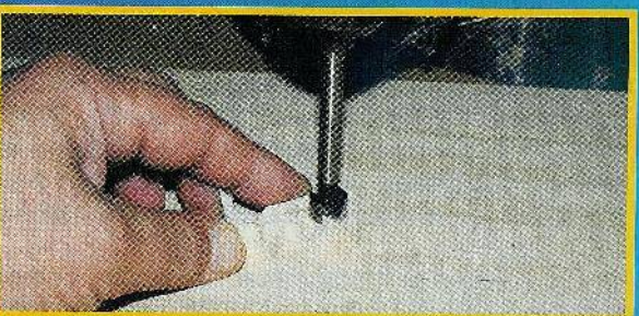
Fig. 7. Using the previously drilled 1/16" hole as a guide, bore a hole 1/8" deep with a 1/2" brad point or Forstner bit.
