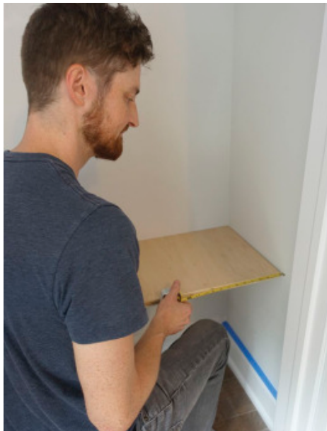
Check the Closet for Square – Use the shelf component itself as a visual aid to tell you exactly how out much you need to trim for a tight fit.
