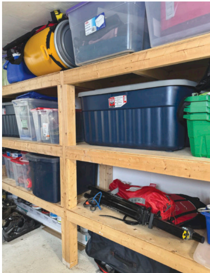
Simple and Strong – Plywood and 2x4s work together to create cost-effective, yet virtually bomb-proof shelving. Large plastic storage bins work in tandem with the shelving to store items of many shapes and sizes. (Photo by Rob Brown)
