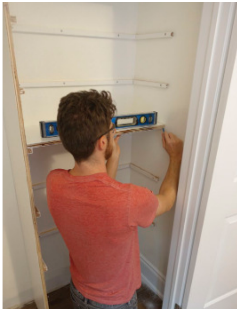
Level Each Shelf – With one cleat installed, Kosonen uses the shelf and a level to mark the location on the opposite side.
