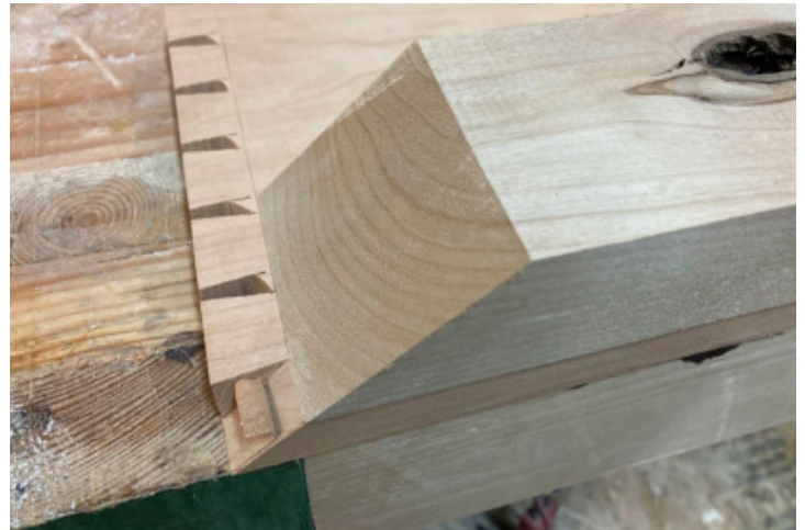
Helping Hand – A mitred piece of scrap, clamped inline with the location of the mitred end of the joint, gives Dobson a guide for his chisel while he's paring the joint.
