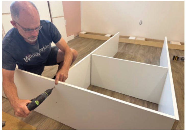
On Its Face – Rest the panels on their faces and attach the fixed shelves, tops and bottoms to them. When everything is assembled, it can be tilted up and into place on the base.
