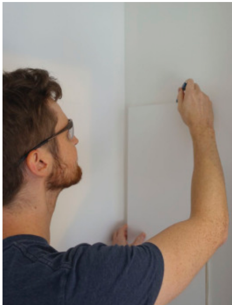
More Accurate Than Measuring – Use the large vertical partition to mark the height that cleats will be installed.
