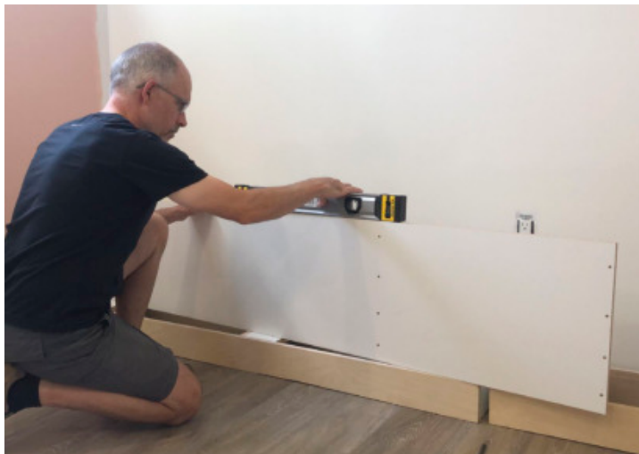
Level It Up – Brown uses one of the longer panels to check the base for square during installation. Notice the pre-drilled holes in the dado and rabbet joints in the panel.
