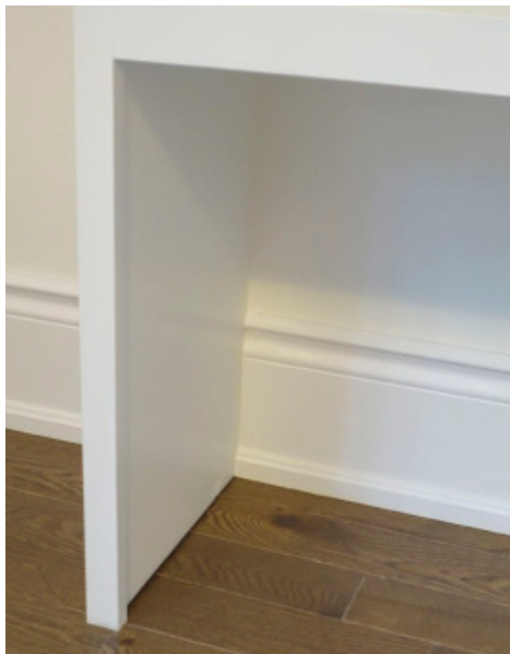
Trim the Baseboard to Fit – Having the baseboard butt up to your shelves gives a finished look.
