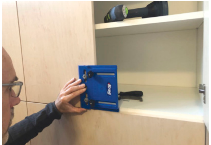
Handle Holes – Brown used a Kreg hardware drilling jig to locate and bore the holes for the handles.
