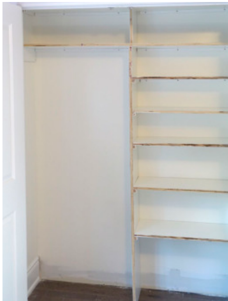
Functional, But Not Pretty – While the shelves may be functional at this point, the face frame provides a finished look.
