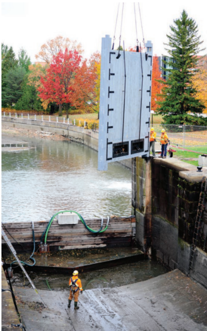
Easier, But Not Easy – Even with today's heavy equipment, installing lock gates isn't an easy job. This was all done by hand 100 years ago.
