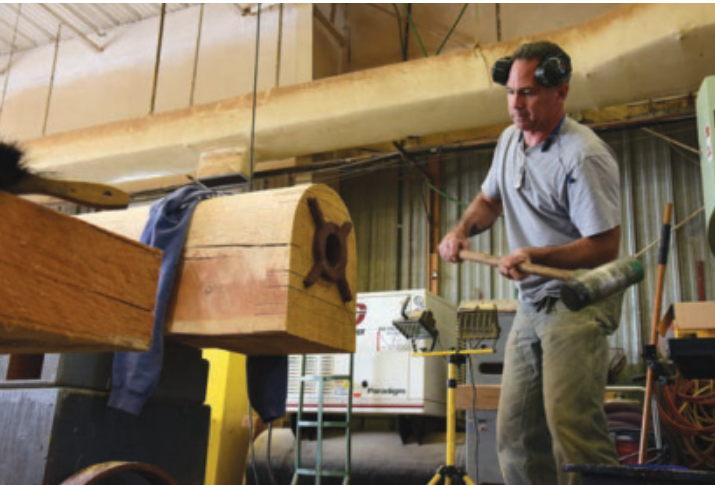
Drive It Home – Using a weighted wooden mallet so he doesn't damage the gudgeon, Matt Churchill drives the steel hinge part home in the mortise that was cut for it.
