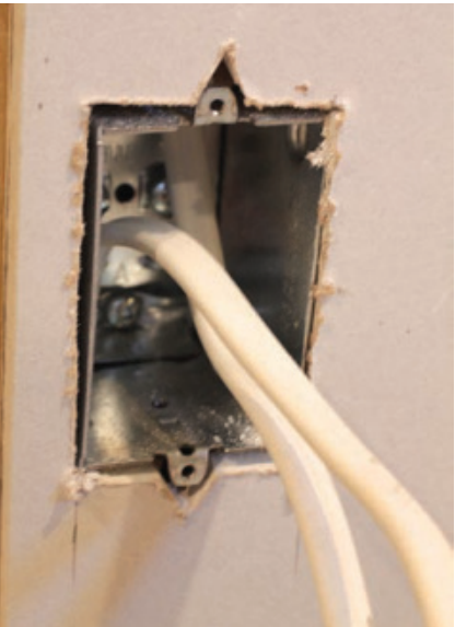
Close, But Not Perfect – When installing drywall you need to be close, but perfection isn't needed. In fact, using tolerances that are too tight can get you into trouble. Any closer around this outlet might have caused the sheet to crack.
