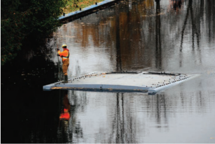
Paddle it Home – Joe Adams poles one of the new gates along the Tay Canal to deliver it to Beveridge's Lock.
