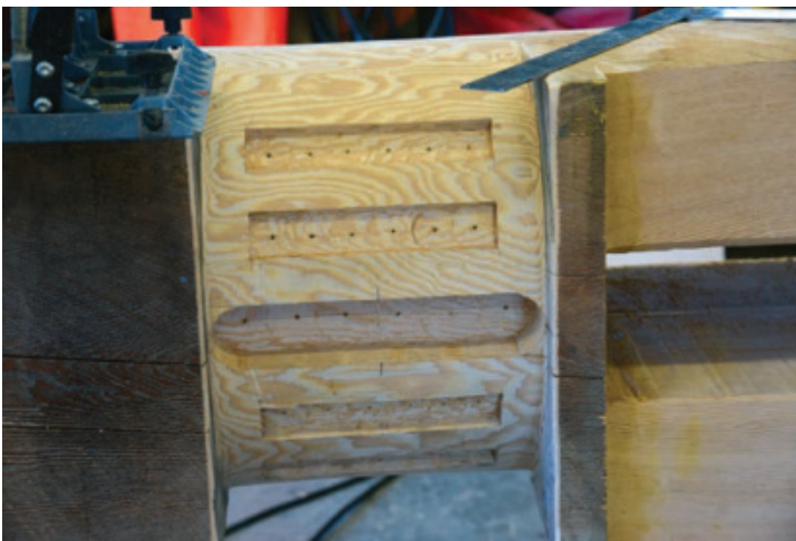
Extended Life – The five wear bar mortises are now complete. When the gate opens and closes the wear bars will dramatically reduce wear on this surface and extend the lifespan of the quoin posts, and therefore the gate.
