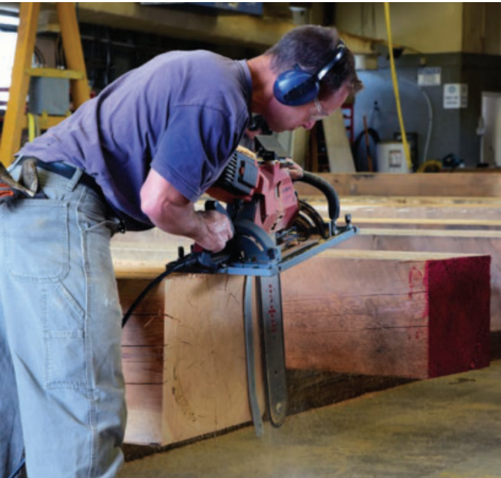
Trimming to Length – Scott Botham uses a Mafell Z6X Ec plunge cut chainsaw to trim the oversized timbers to finished length.
