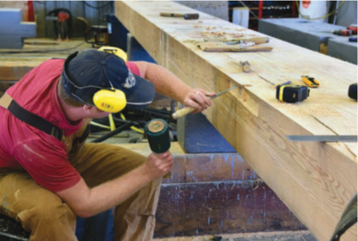
Hand Tools Are Flexible – Hand tools, like when used to build furniture, are very flexible. Here, Joe Adams cuts the mortises to accept the metal railing stations in the top of the gates. These are fastened in place with galvanized bolts.
