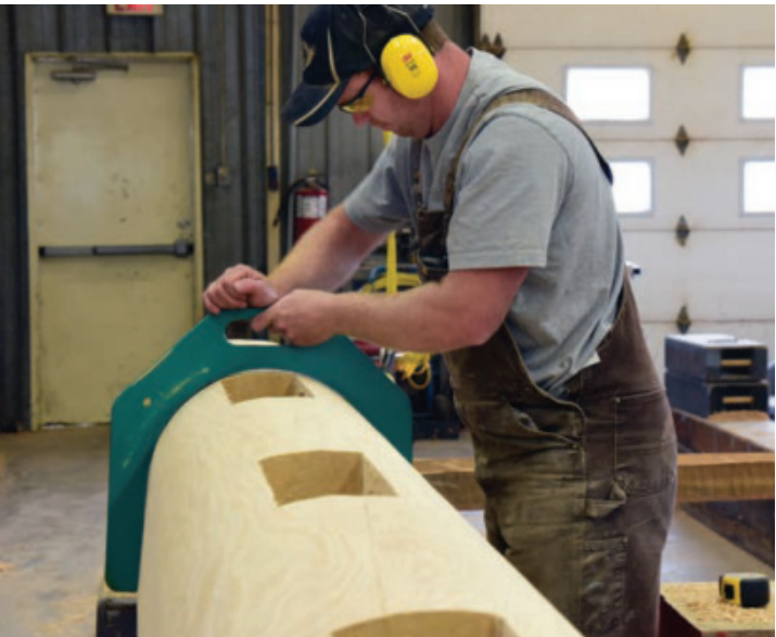
Templates to the Rescue – A template is used to check the shape of the quoin post while it’s being brought down to its final shape. Much of the work done in the shop is repetitive, so templates are used to speed the process and work more accurately.
