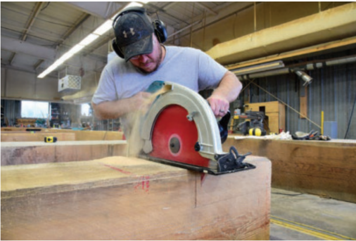
Huge Tenons – Josh Bennett begins the cuts to make the huge tenons on the ends of the gate rails. These are the main joints that keep the gates together.
