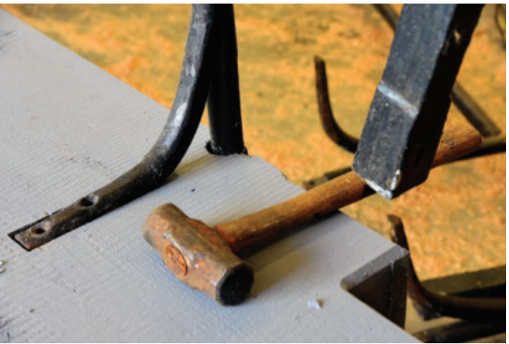
Final Pieces of Hardware – The steel safety rail is being installed in the hand cut mortises on the gate top.
