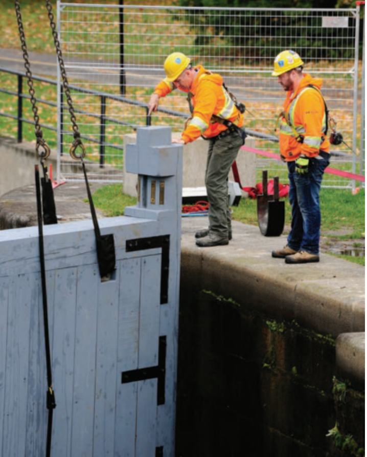
Final Resting Place – Matt Churchill and Josh Bennett drop one arm of the Beveridge's Lock gate into place.
