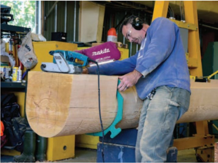
Sanded to Perfection – Matt Churchill checks the dimensions of the band mortise in the quoin post with a template. The fit gets adjusted with a belt sander equipped with a coarse grit belt.
