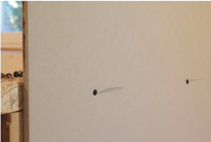
A Few Pencil Marks – Adding a few pencil marks to a piece of drywall before it goes up will go a long way in helping you get the first few screws in place to secure the sheet. This is especially true when working alone.
