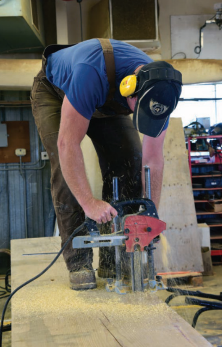
Take the Plunge – The openings for the gate valves are made with a plunge cut chainsaw.
