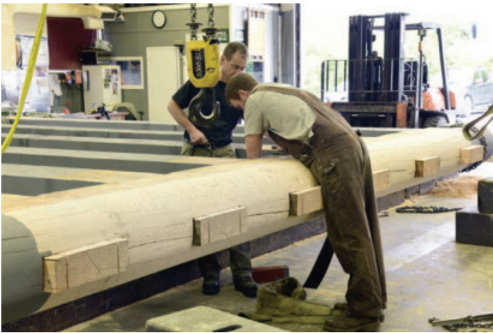
Chains for Assembly – Here, the crew positions the chains they will use to bring the gate together.
