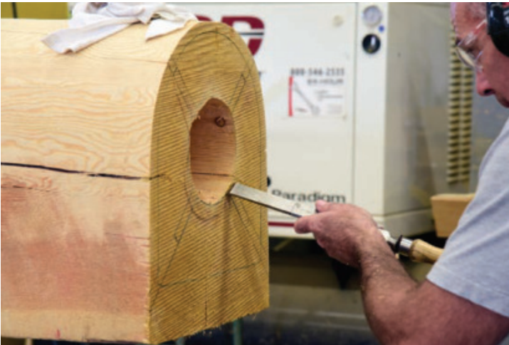
Make Way – Waste from the centre section of the quoin post, where the steel gudgeon will fit, is removed with a 1-1/2" framing chisel.
