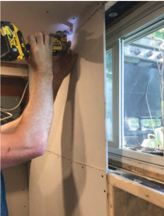
Trim After – Installing a sheet of drywall, then cutting the window and door openings, is often the easiest approach. There's a much lower chance something will go wrong this way, whether that's the sheet breaking during installation or you cutting the opening in the wrong location.
