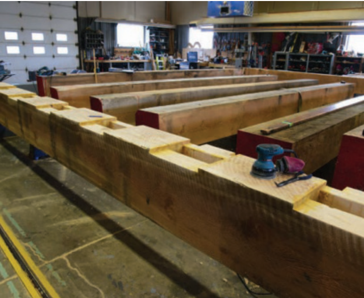
Quoin Post – The mortises are laid out on the quoin post and are lined up to accommodate the tenons in the rails, which still have to be cut.
