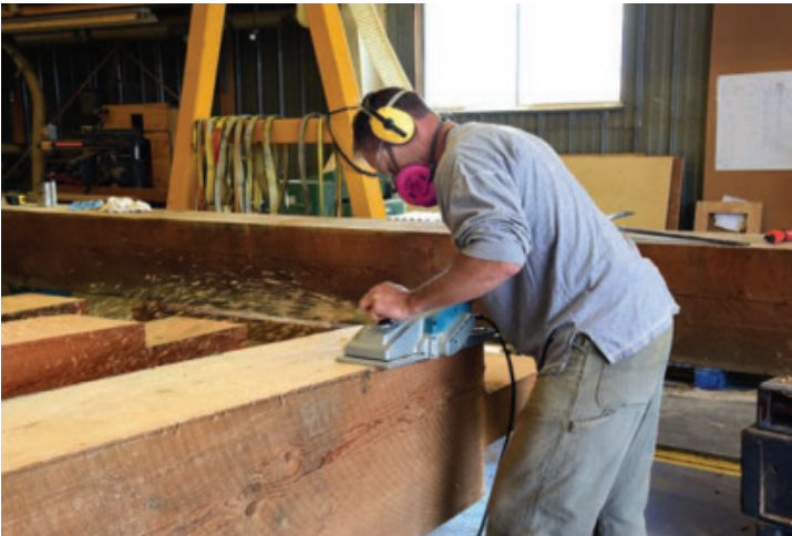
Final Shaping – The final shaping of the cambered rail faces is done with a powered hand planer.
