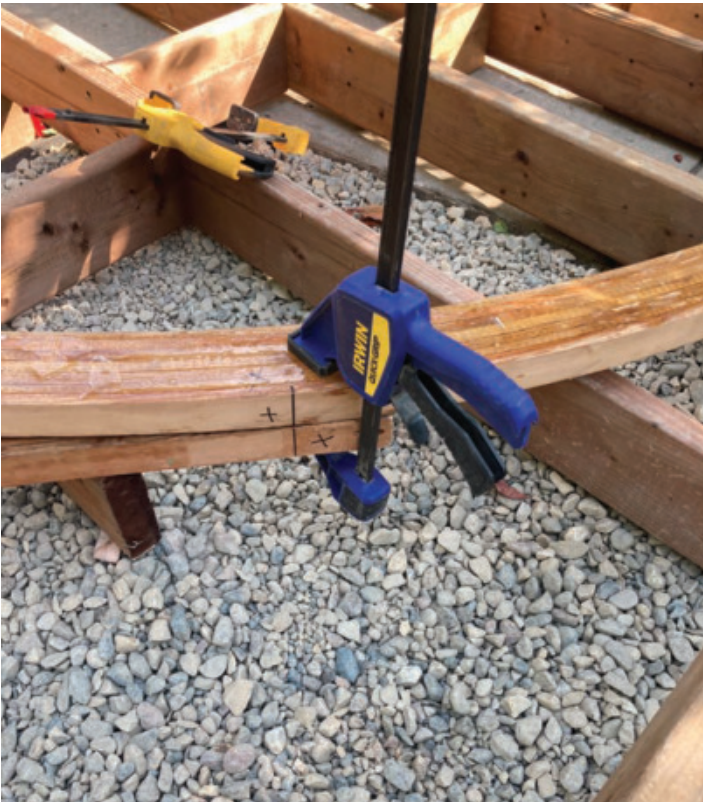
Cut to Length – With the epoxy dry, Jensen brought the three wave-edge laminations to the deck to mark where they would be trimmed to length.
