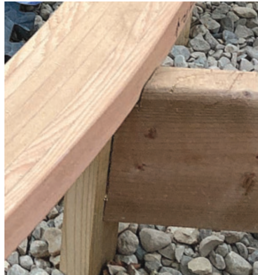
Notched Out – The deck boards are thinner than the wave edge, so Jensen had to notch the joists to accept the wave edge. Since slight variations can occur between the joists, he cut the notches about 1/8" deeper than needed so a customized shim could be used to account for any variations.
