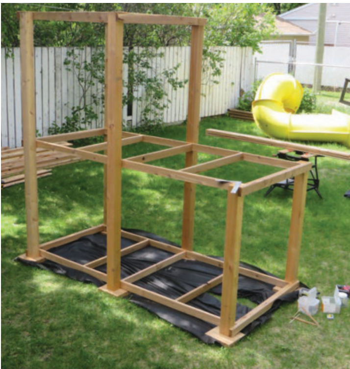
Start Towards the Outside – Chemerika started with the 4' × 8' perimeter and fixed the corners in place with 4×4 posts. Adding intermediate 4 × 4s and a few more structural components, and the basic shape started to be visible.
