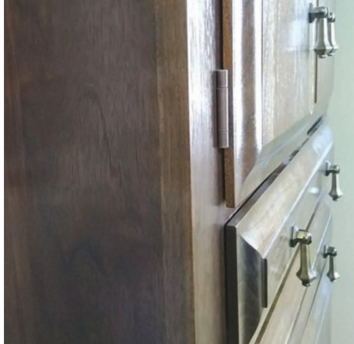
Invisible Joints – The glue line where the face joins the sides of this armoire is rather obvious, and not very pleasing to the eye. A lock mitre joint will remove this problem.
