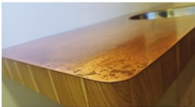
Patina – Splash-effect patina is easily created with vinegar and salt. Play around with some copper offcuts before using the real thing.
