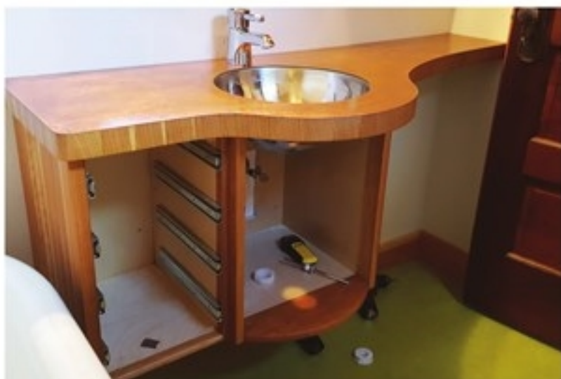
Install Cabinets and Countertop – Installing the faucet before the countertop is often easier.
