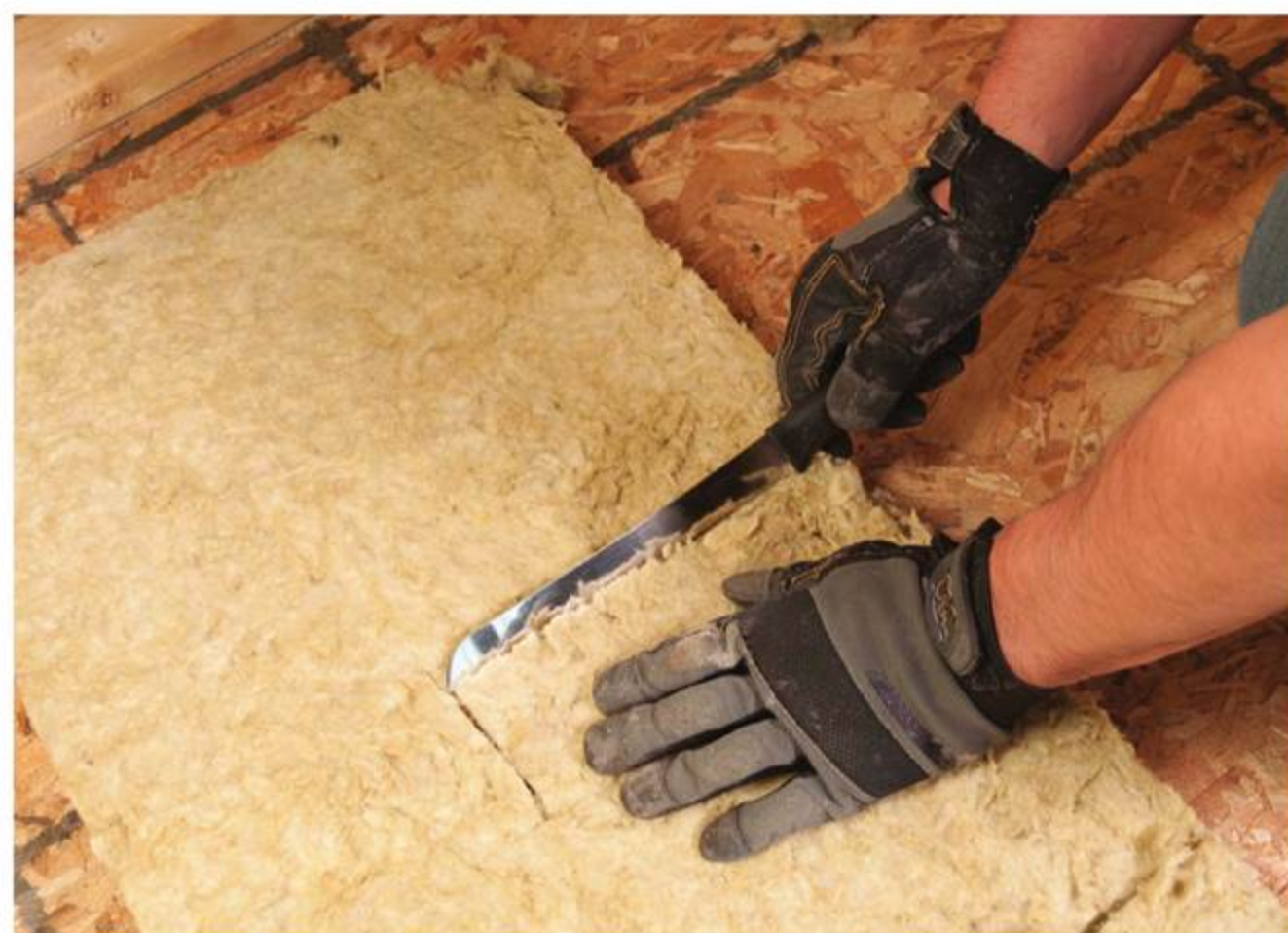
Premium Batts – Rock wool is stiffer than fibreglass, and can be easier to handle and install. It's easily cut with a knife. (Photo by Roxul)
