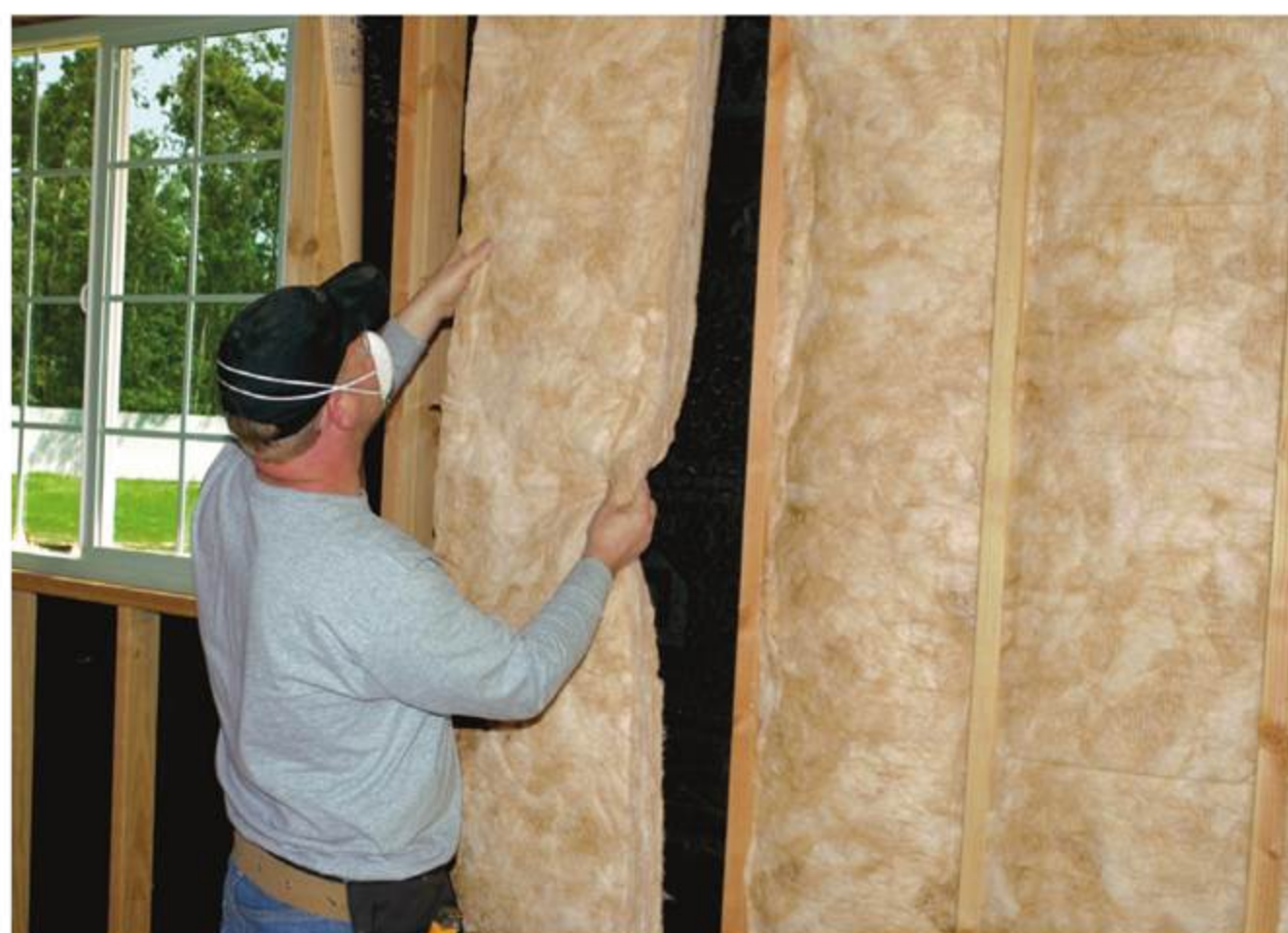
Fiberglass Batts – The most commonly used type of insulation in Canada, fiberglass batts are an economical choice and are fairly easy to install. (Photo by CertainTeed)
