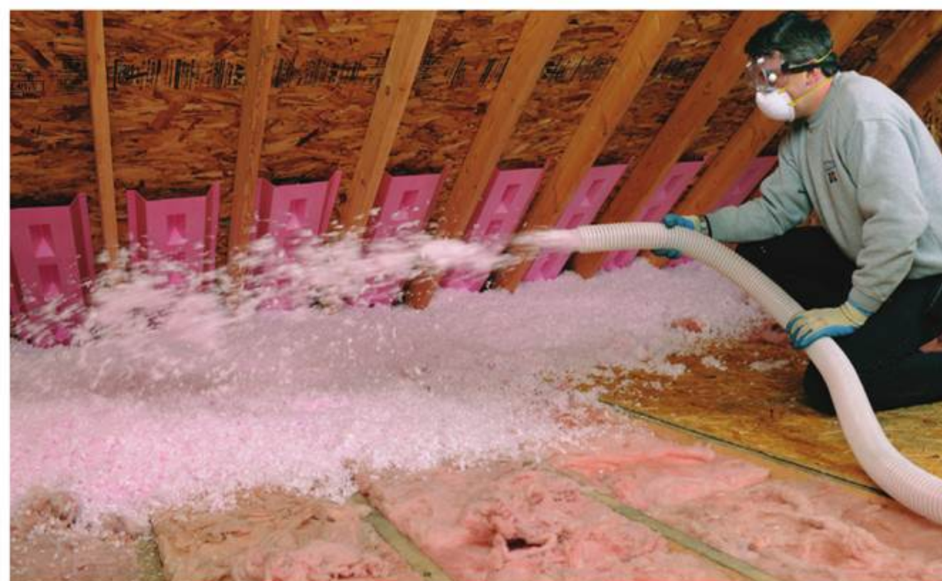
Blow It in Place – Blowing fibreglass or rock wool insulation into an area can be very efficient, though a helper is needed to feed the hopper. (Photo by Owens Corning)
