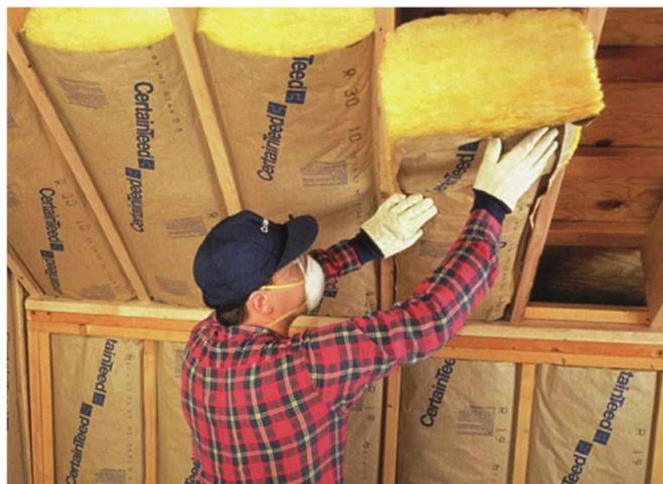
Vapour Retarder – A Kraft paper or foil vapour retarder is sometimes attached to one side of fiberglass batts. (Photo by CertainTeed)
