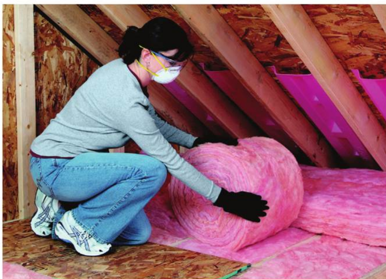
Rolled Fibreglass Insulation – Rolls of fibreglass insulation are available in long and wide dimensions, and are great for covering large, flat areas. (Photo by Owens Corning)
