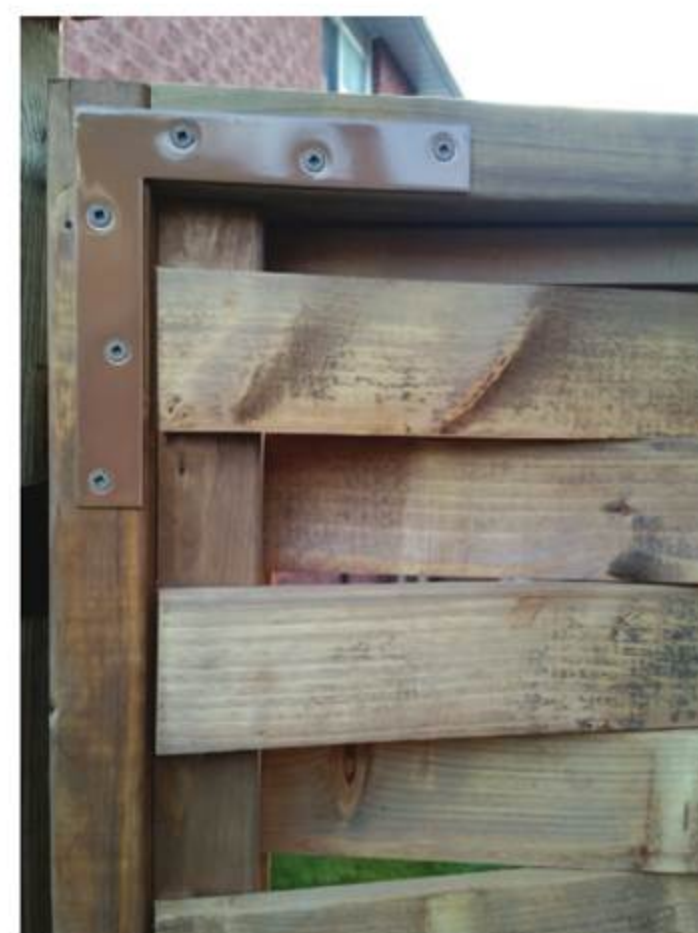
Face Frame – Mitre the ends of the face frame so they meet right at the corners of the main frame.
