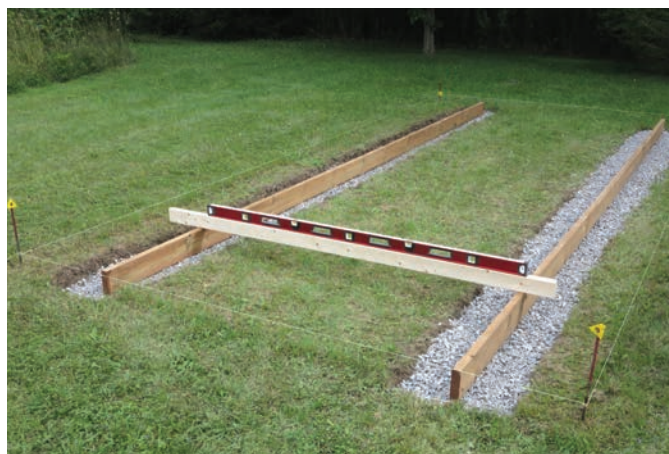
Level it Out – By using future rim joists and a spirit level you can assure the beds are flat and level.
