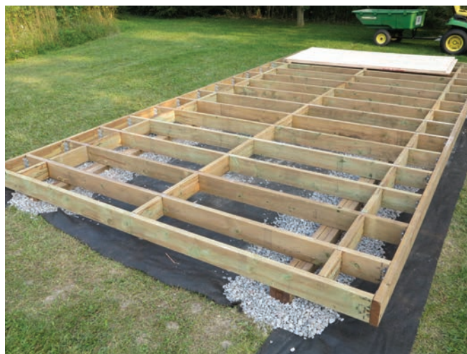
Ready for Flooring – With the joists spanning the skids, and capped by the rim joists, you can add blocking, joist hangers and landscape cloth.
