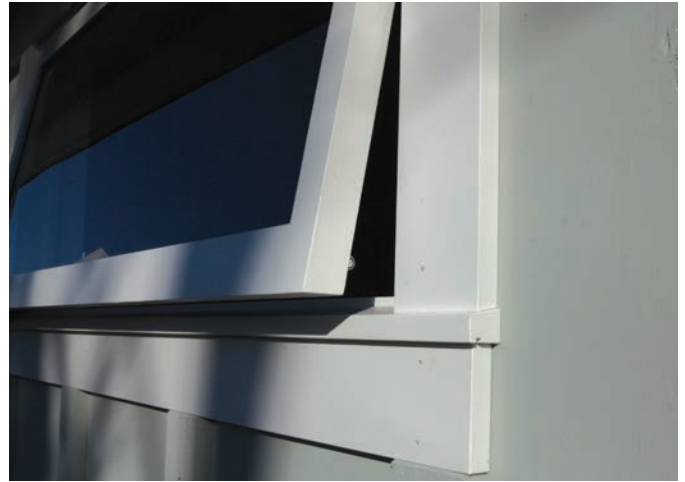
Window Details – Once the window trim is secured in place you can see how the sill extensions play into the overall look. Notice the drip edge under the sill.
