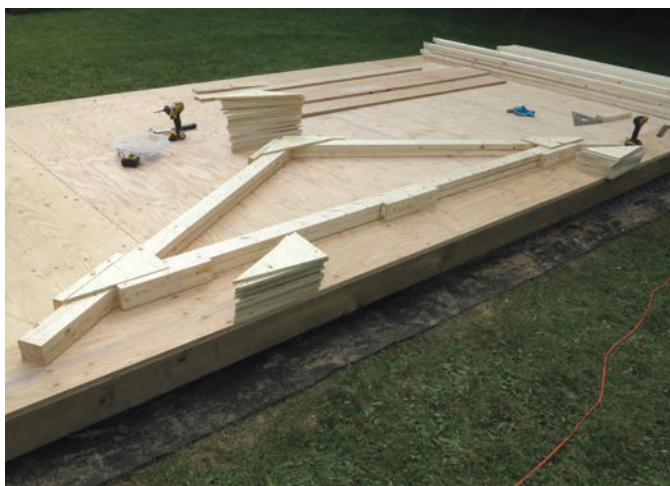
Truss Jig – Salusbury laid the floor, then set up some blocking to assist with assembling the trusses. Here, the first truss is ready to be removed.
