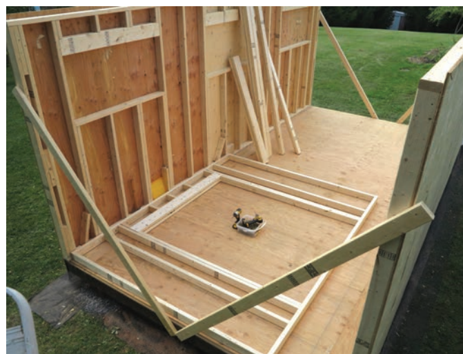
Second Wall – With the second wall built in two sections it can be positioned and screwed in place. Screws through cladding draw this wall tight to the rim-joists. Notice the third wall on the floor, ready to be erected.
