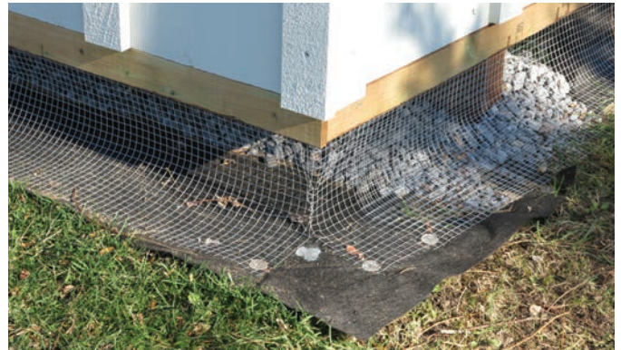
No Critters – Critter screening allows airflow, but deters unwanted occupants.
