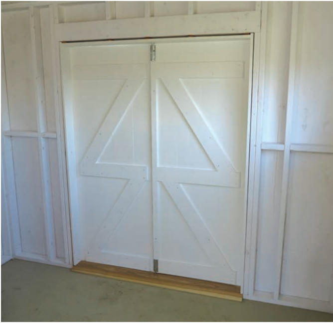
Installed Doors – Nicely fitting doors are installed and ready for use.
