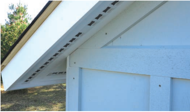
Gable Ends – Gable detail, showing soffits and rough-sawn trim and battens stained to match the cladding. Notice the angled edge of the horizontal member, aiding in water runoff.
