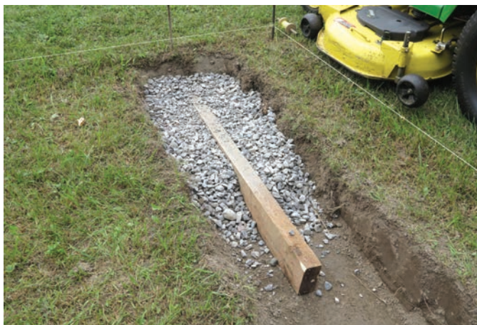
The Right Depth – A moveable 4" wide board helps you to gauge the depth of stone.
