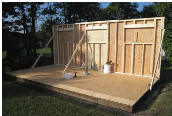
The First Wall – Once it was built in three sections, and erected, Salusbury joined them together and braced them.
