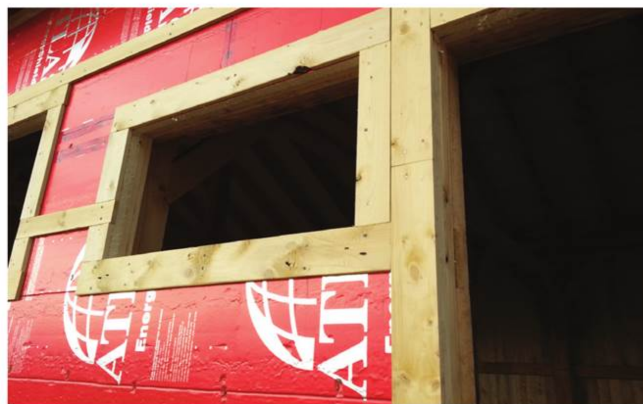
Rough Openings – Window, door flanges and trim require nailing all the way around an opening.
