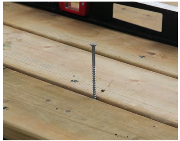
Details are Important – Small details like leaving minimal spacing between decking (less than 1/4") will make for a much more wheelchair-friendly ramp. A screw makes a good spacer.
