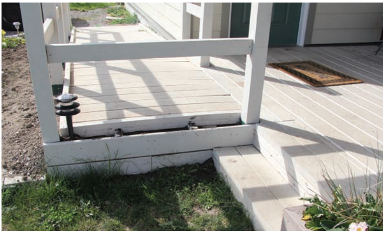
Low Maintenance – Durable materials such as the composite decking on this access ramp will ensure a long life and require very little maintenance.
