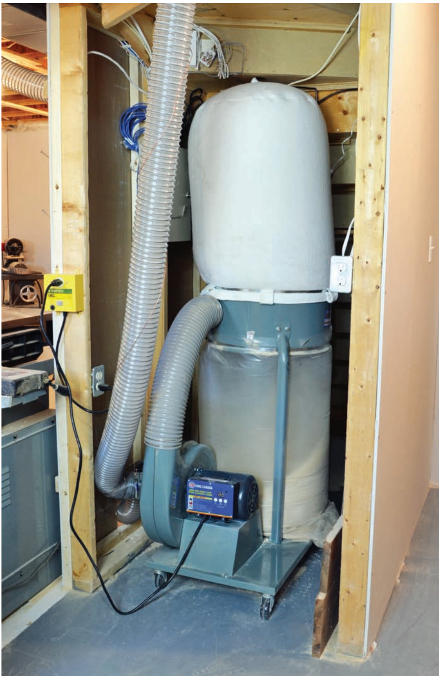
Dead Space — Brown used the area under his stairway to store his dust collector. It was otherwise wasted space. Notice the iVACPro system to the left of the collector, simplifying dust collection.
