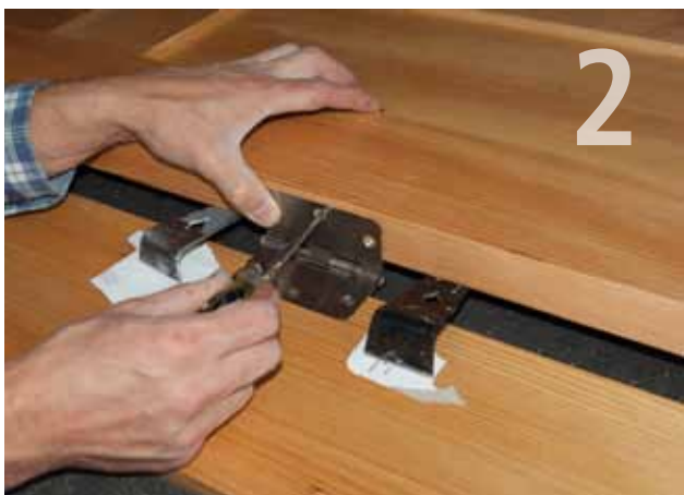
Lay the Door Down – Attach the hinges to the jamb, then the door. Double-check that you're installing the hinges so the door swings correctly.
