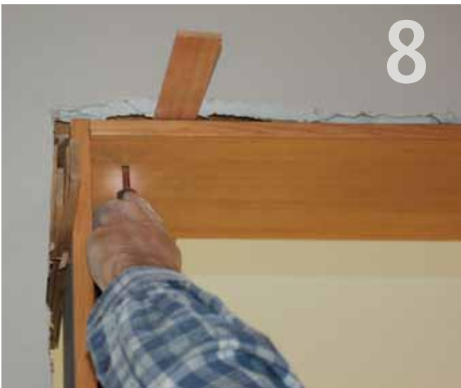
Reach Up – If you need to, use a 3" screw to adjust the head jamb. You just want the gaps on the hinge side of the door and the head jamb side of the door to be equal.
