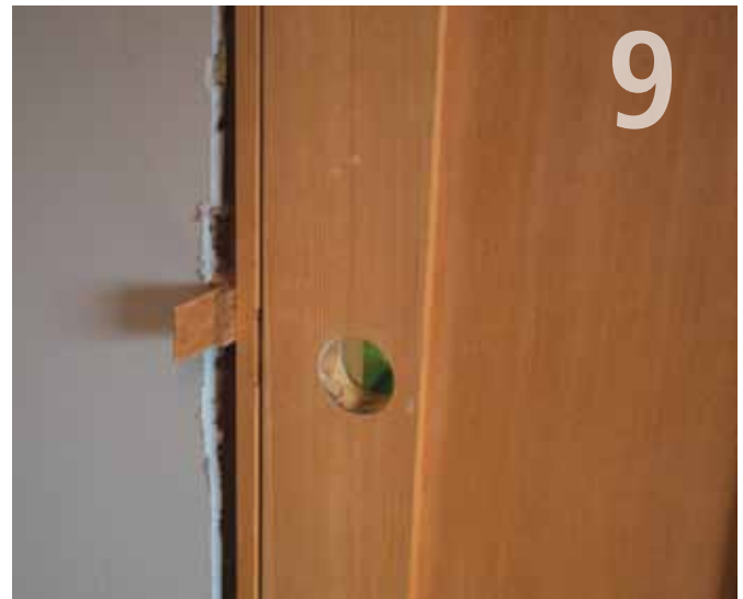
A Strong Latch – When securing the latch side of the jamb, install shims that mirror the hinge side and take extra care to shim the area around the door latch.
