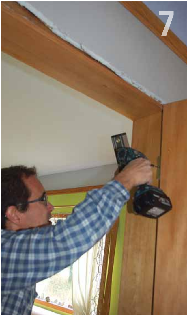
Hinge Side First – Secure the hinge side of the jamb with 3" #8 screws. The screws will be covered by the door stop.
