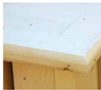
Clean and Tidy – A mitre joint finishes off the decking ends. The decking ends help protect the decking boards.
