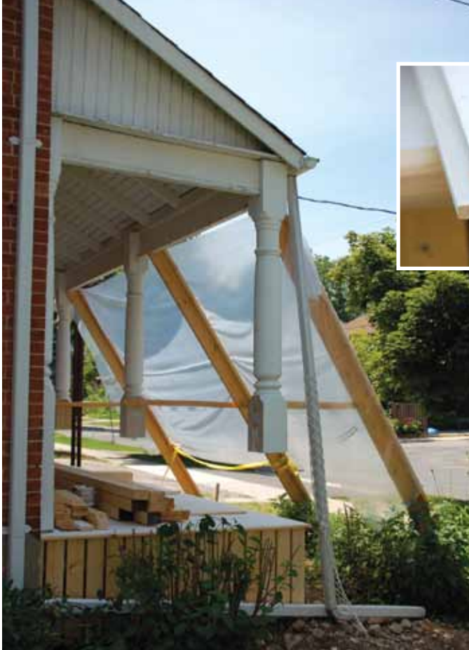
Helping Hand – While the decking was removed, supports did the heavy lifting, supporting the porch roof.
