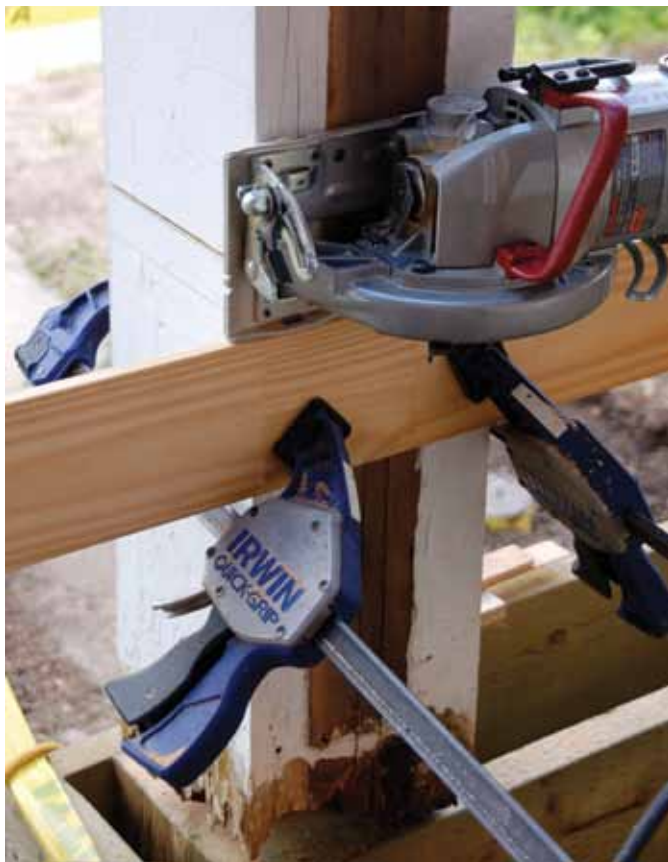
Remove the Rotten Wood – Dunkin used a straightedge to guide his circular saw as he made cuts around the perimeter of the post. Once the saw did its job, Dunkin grabbed a handsaw and finished removing the rotten section of wood.
