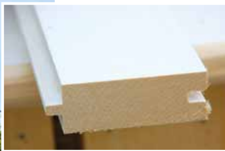
Prime Then Install – The 5/4 pine decking was primed before installation to protect it from the elements, and prolong the life of the deck.
