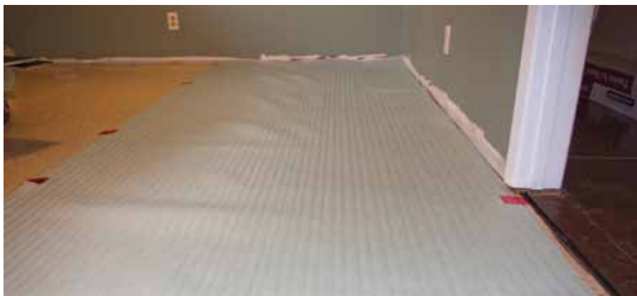
Add Underlay – Install underlay before laying any boards. It should go right up to the walls, and can be taped down.
