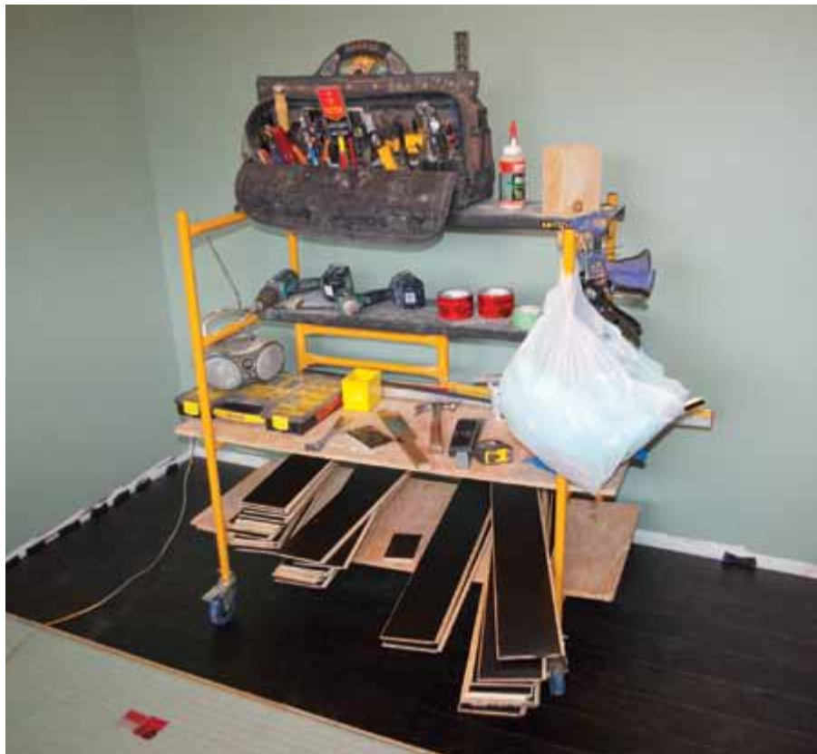
A Helping Hand – Kinzel uses a rolling cart to keep his tools from damaging the newly laid floor but still have easy access to them. The cart also ensures he doesn't trip over tools and materials – a frustrating and dangerous occurrence.
