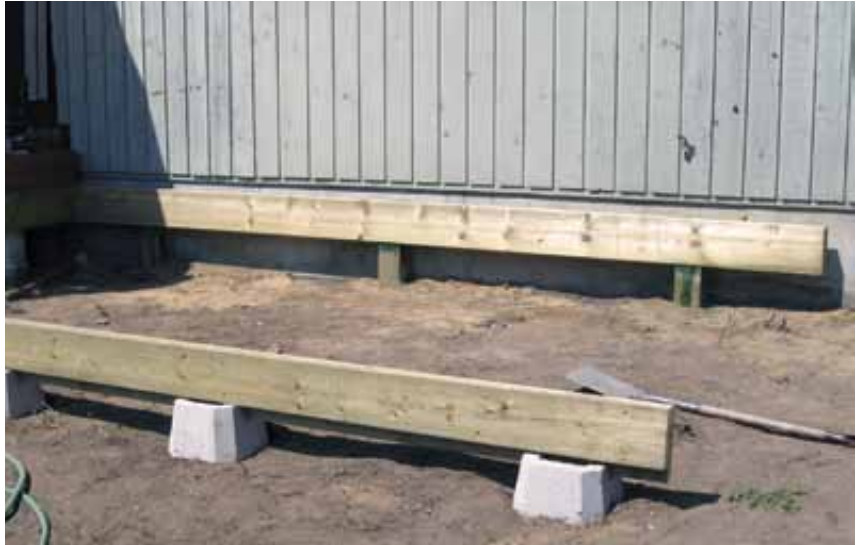
Block Footings – Dig properly sized holes and fill them in with care to give block footings a stable hold.
