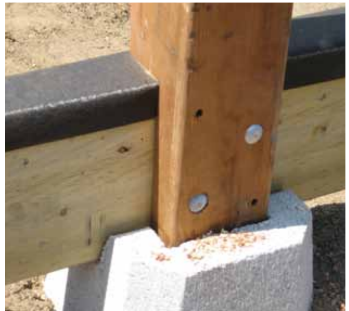
Please ... Overdo it – When laying the beams Shervill recommends to either increase the width of each beam or the quantity of beams to provide a solid platform to build on.
