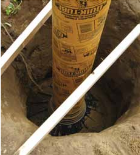
Dig Deep – A deeper hole and bell footings on the bottom of your forms provide a rock solid foundation.
