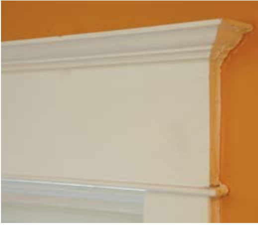
Details Are Important – Detail of existing trim that needs to be matched.
