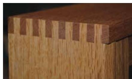
Super strong – Finger joints provide a very strong corner connection for cabinets and boxes.
