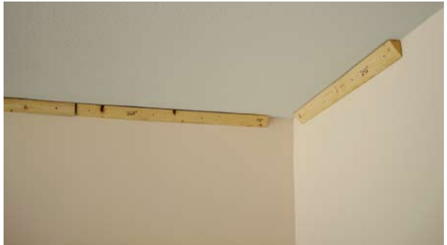
Solid surface – Nailing strips give you a dependable nailing surface onto which the crown can be secured.
