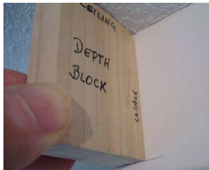
Mark the depth – The use of a depth block will make it easy to mark the crown location. Avoid chalk lines because they can be quite messy.
