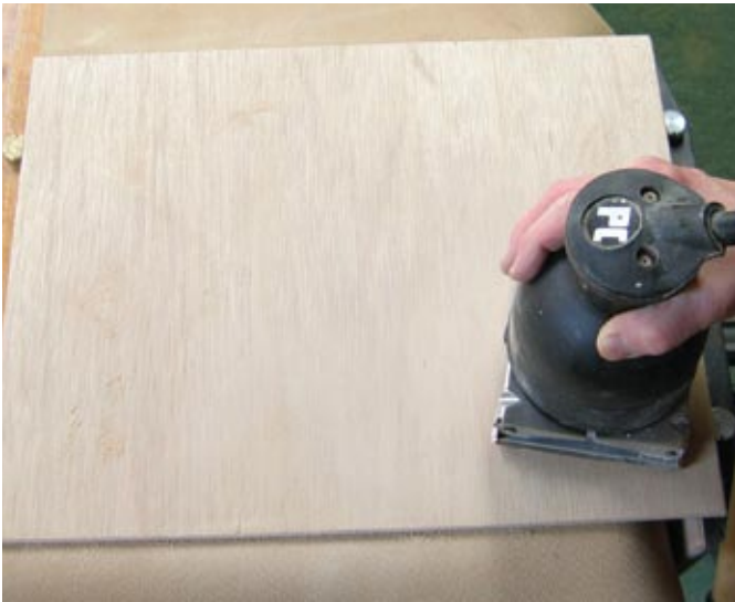
Prepare the panel – Sand the panels starting at 100 grit through to 220 grit.
