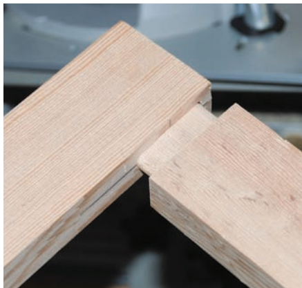
Perfect mortise and tenon joint
