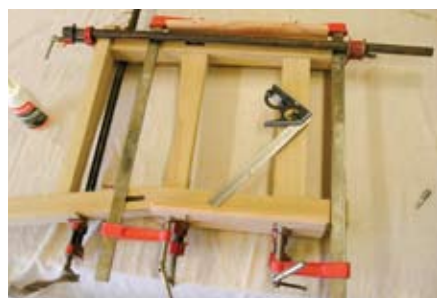
Gluing up side assembly
