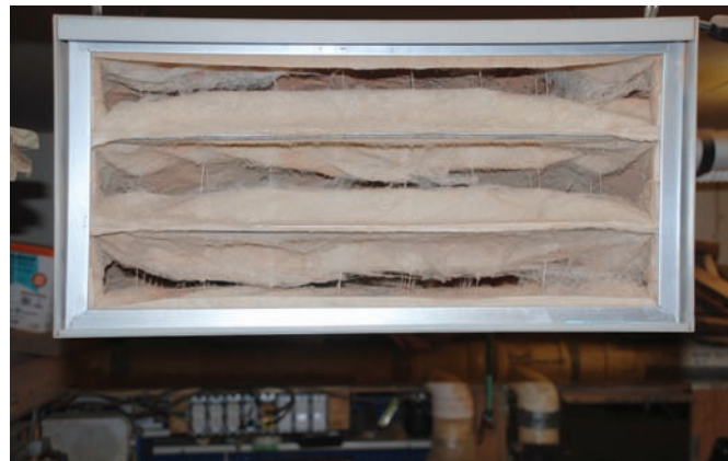
Bag filter inflated and cleaned
