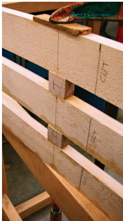
Laminations with spacers F installed
