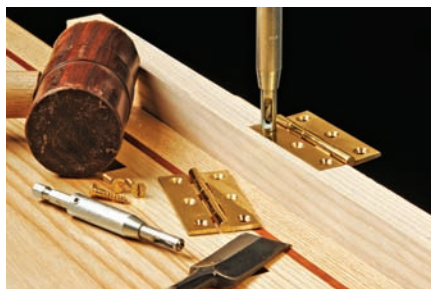
Use centering bit to drill holes
