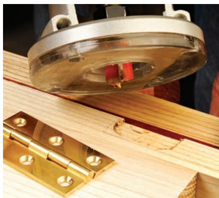
Cutting mortise with a router
