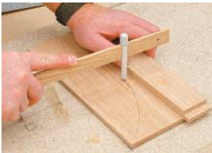
Mark out the hutch door arches
