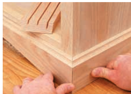
Install the base skirt
