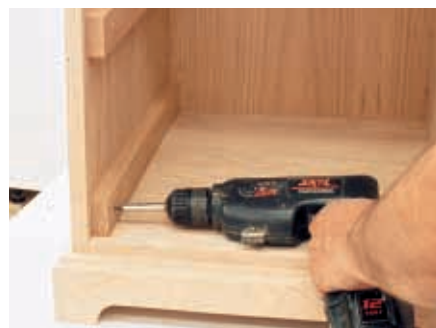
Screw in three space cleats
