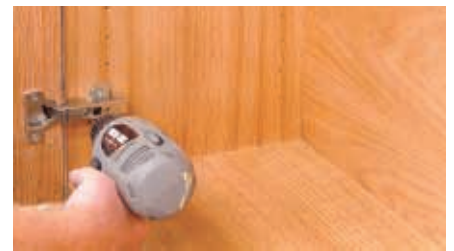
Clip hinge plate on hinges and install doors
