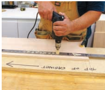
Drill two columns of holes in each side panel for shelf pins
