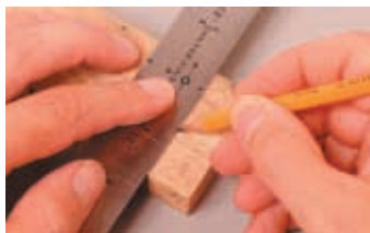
Lay out tenon on end of stock
