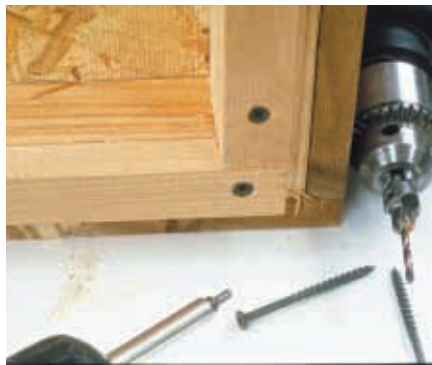
Cut base strips and attach to bottom frame
