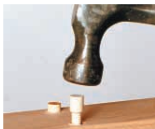
Hammering Miller Dowel
