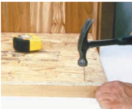
Cut and attach bottom board
