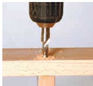
Drilling for Miller Dowel
