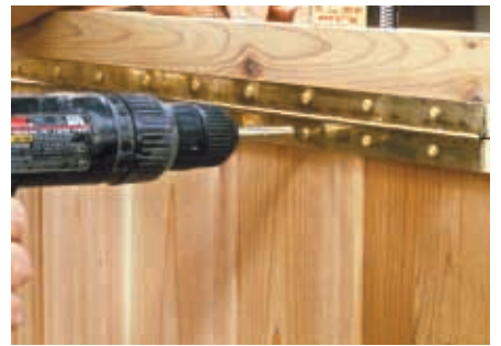
Attach brass piano hinge
