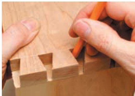
Position tails on the end of the matching board and mark pins
