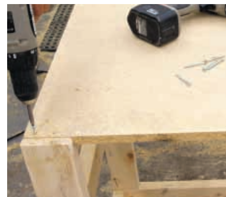
Glue and screw bottom board into leg rabbets
