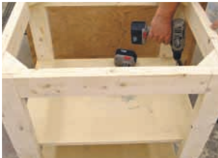
Attach middle board with screws
