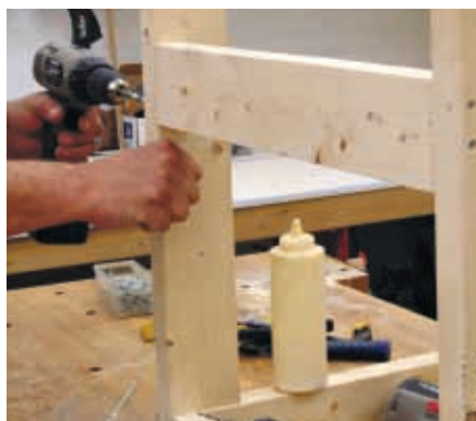
Attach support rails to frames with butt joint and glue
