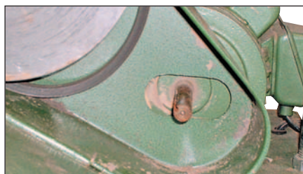
Large oblong opening needs seal
