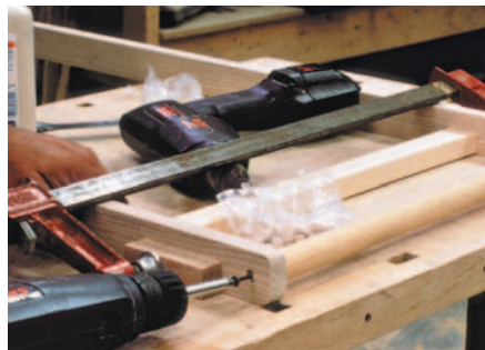
Inset rod into rail holes
