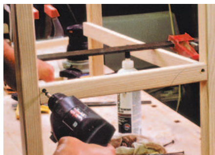
Install lower cross rails
