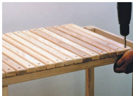
Install slats with 1/4" spacing and 1/4" overhang
