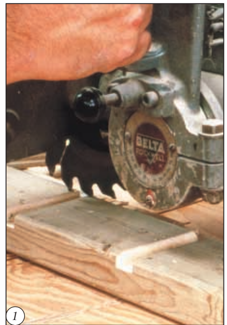
Cut grooves in uprights
