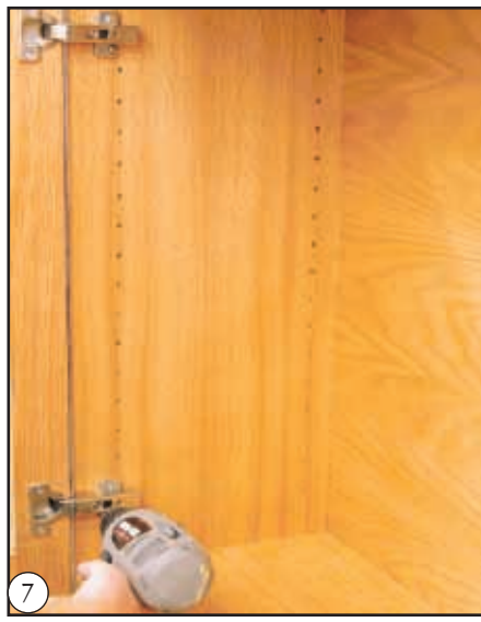
7 Drill hinge holes
