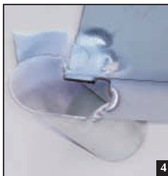
Inside of lower door with pipe and enclosure shield pieces in place.
