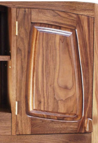
Pic.2 The door looks more complex than it is. All the joints are 'straight' but they are offset on the outer (meeting) stile
