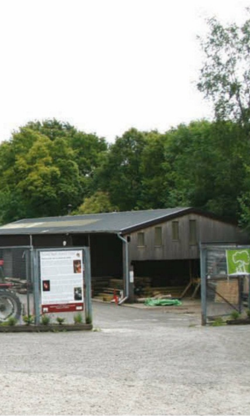
Sheffield The Eccleshall Project in Sheffield provides workspace for craftspeople (left), a gallery to display their work and sells timber on site
