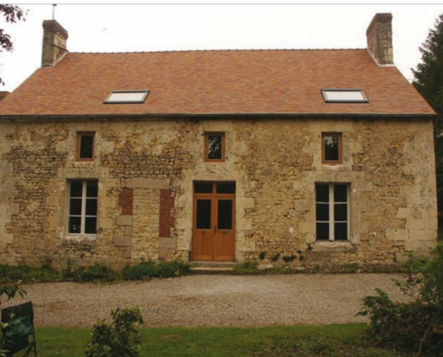
Longère One of Gordon's most recent commissions was to make new oak doors for a longère in Normandy, replacing the old single door with a pair, plus fan lights above
