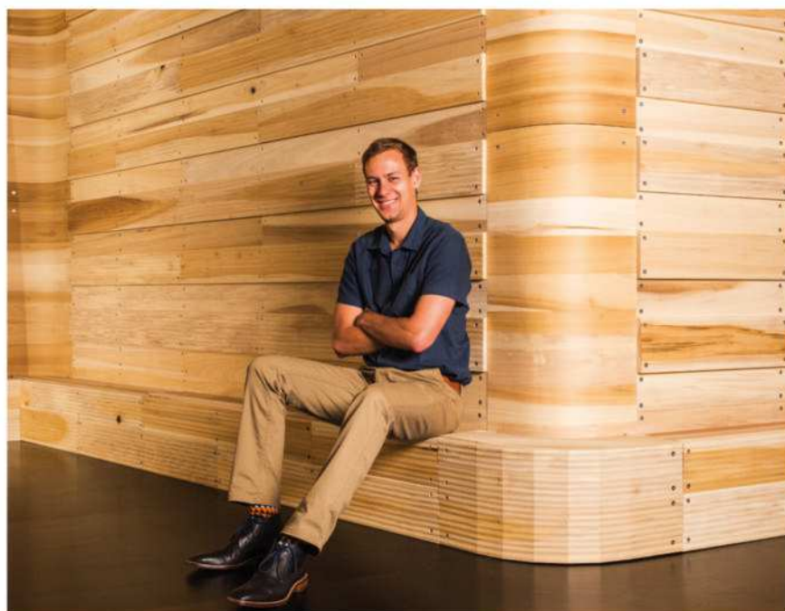
Below: American tulipwood acoustic wall for the Northern Beaches Secondary College Performance theatre. Photo: Jack Bussell
