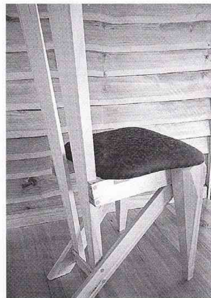
Above: Lining boards and furniture made from radially sawn timber.
