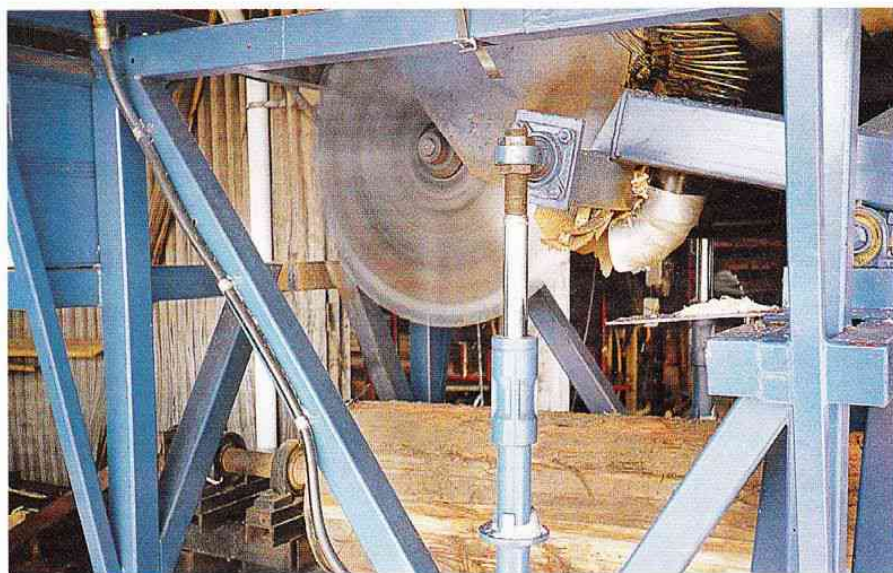
Sawblade ready to be lowered for the first cut.
