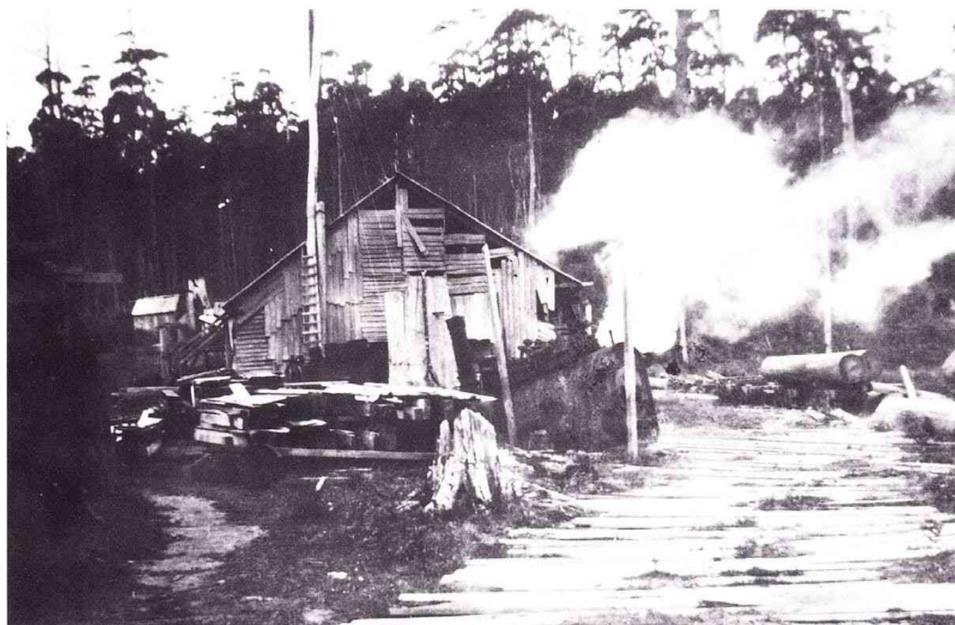
Britton Bros.' steam driven mill at Britton's Swamp in Smithton, Tasmania in the mid-1930s. The board track in the foreground was for early model log trucks to deliver logs to the mill. Tramlines were used for the transport of logs to the mill and also to push timber trolleys to the stacking bays. The mill cut mainly blackwood and Tas. oak sourced from State Forest leases in the Brittons Swamp area. Photo courtesy Britton Bros. Pty Ltd.
