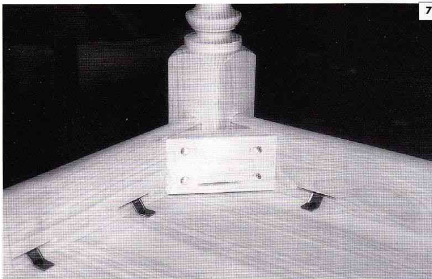
Top and frame secured with screws and steel clips. Note glue block with four screws and glue.
