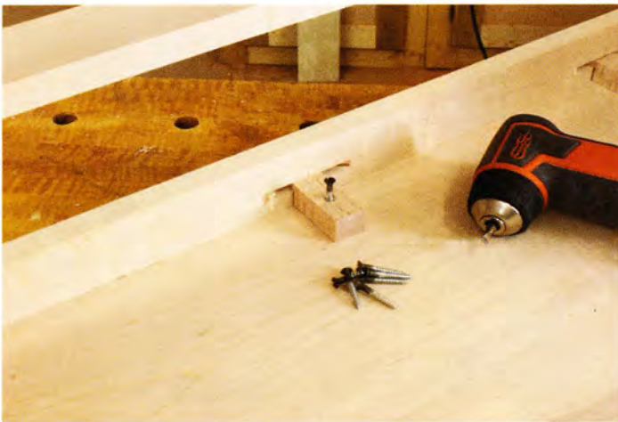
24 Join the top to the case. To allow for seasonal movement, use wooden clips and #8 x 1\frac{1}{4} " screws with the heads blacked for aesthetics.
