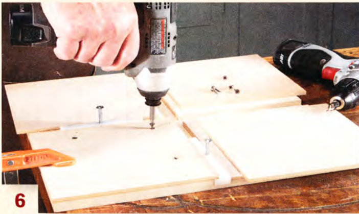
6 Put the sliders in the base's grooves, then trap them with four square pieces of 1/4" plywood. Fasten these pieces to the base.
