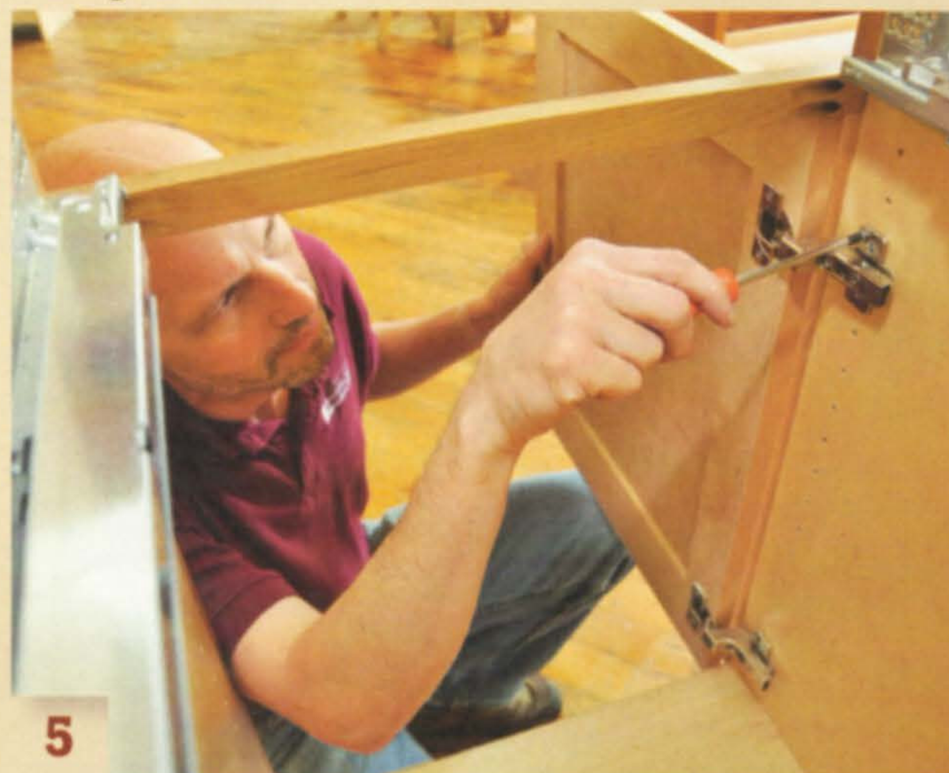
Mount the door by clipping the hinge cup arms onto the hinge plates. Then use the adjustment screws on each hinge to center the door in the opening and make it flush with the face frame.
