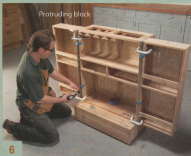
6 Install the doors. Clamp each one to the cabinet, flush at the top, with blocks protruding beyond the inside edges. Press the open hinges against the blocks as you install the screws.
