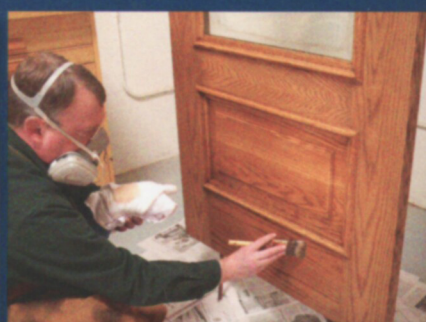
Finish An Exterior Door 5 Essential Steps
