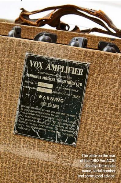
The plate on the rear of this 1962 Vox AC30 displays the model name, serial number and some good advice!
