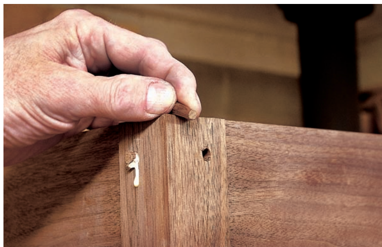
Split out the pegs. Then shave them to size with a paring chisel.
