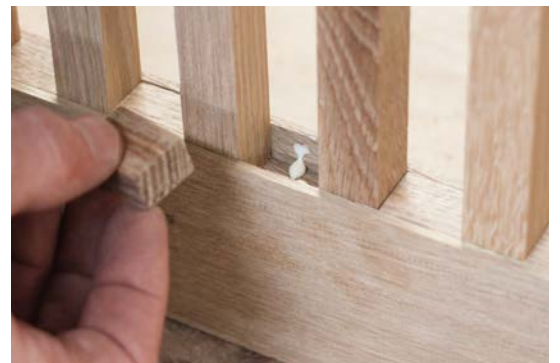
A DROP OF GLUE WILL DO. Hold the spacers in place with a small drop of glue. Don't glue the spindles. You can also use a 18-gauge nailer to tack these pieces in place.
